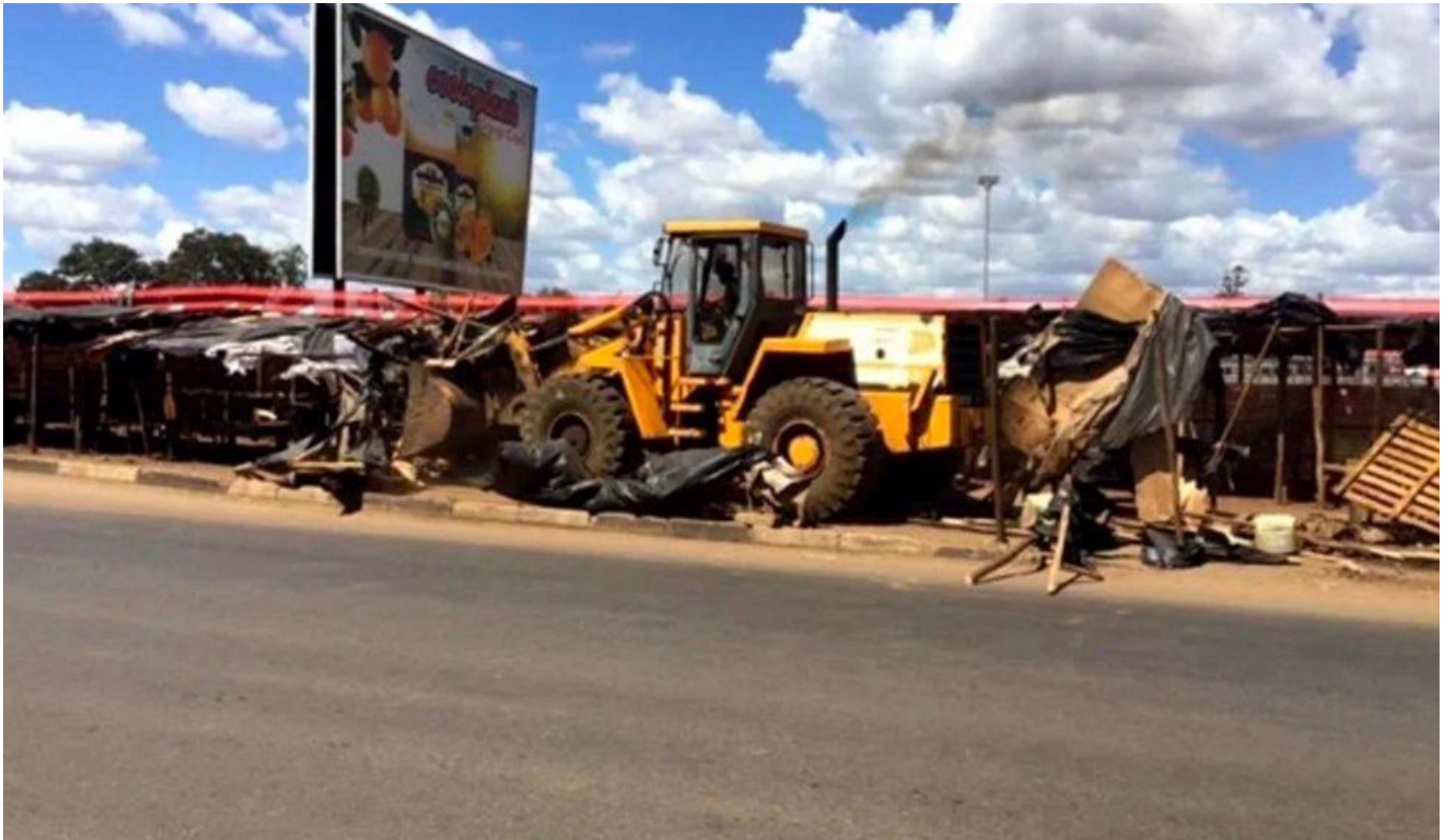
Demolition of informal sector operating spaces in Mbare
