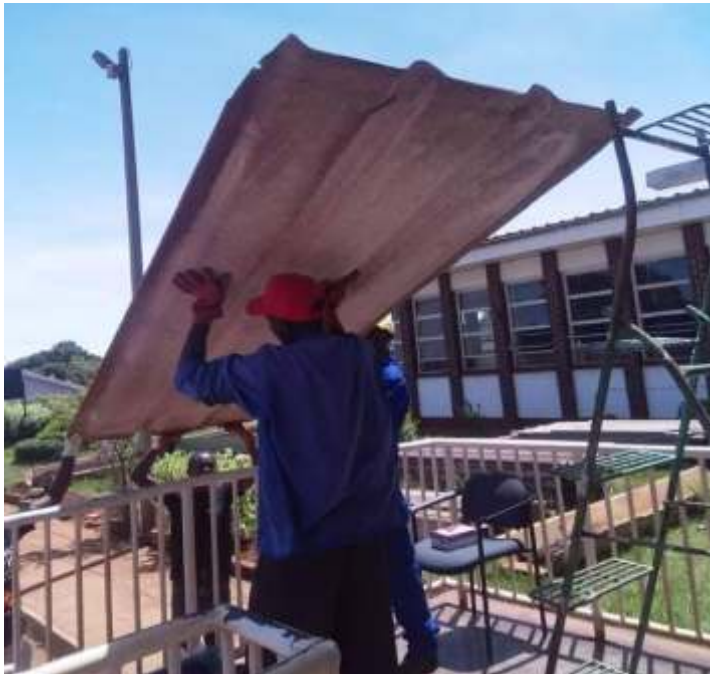
Men At Work At The Hatcliffe Clinic Maternity Ward Roof
